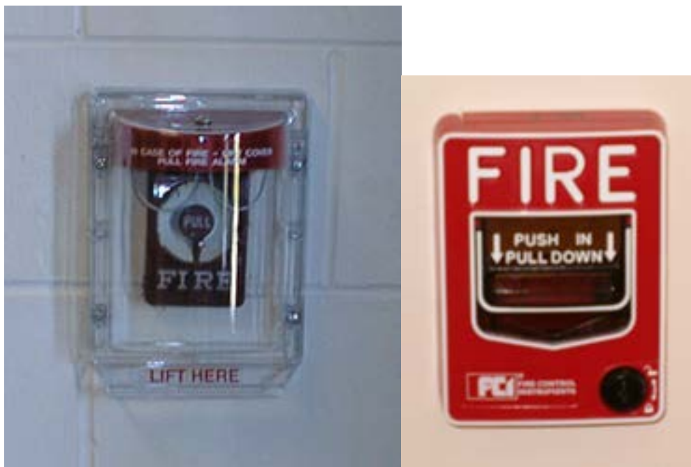
Manual Pull Stations with Plexiglas cover and without
